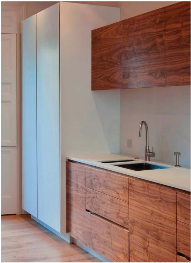
Full height white units with Corian® clad plywood doors with Corian® external trims, panels and cladding by Jack Trench Ltd.
