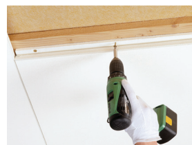
Master F is installed by screw fixing
