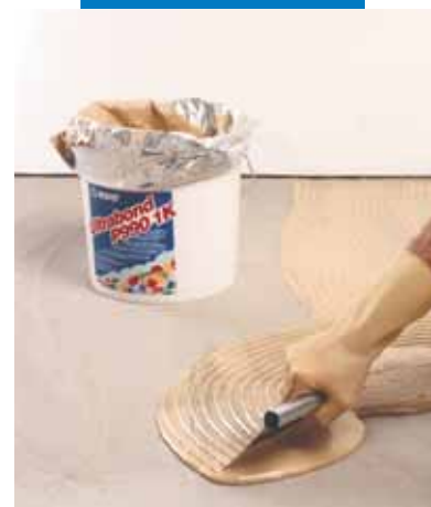
Spreading the adhesive
