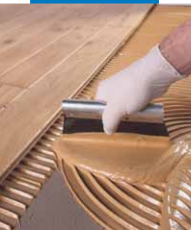
Spreading Ultrabond P990 1K
