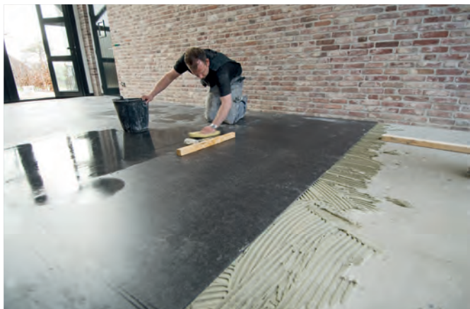
12 Grouting and cleaning 12 Rejuntado y limpieza
