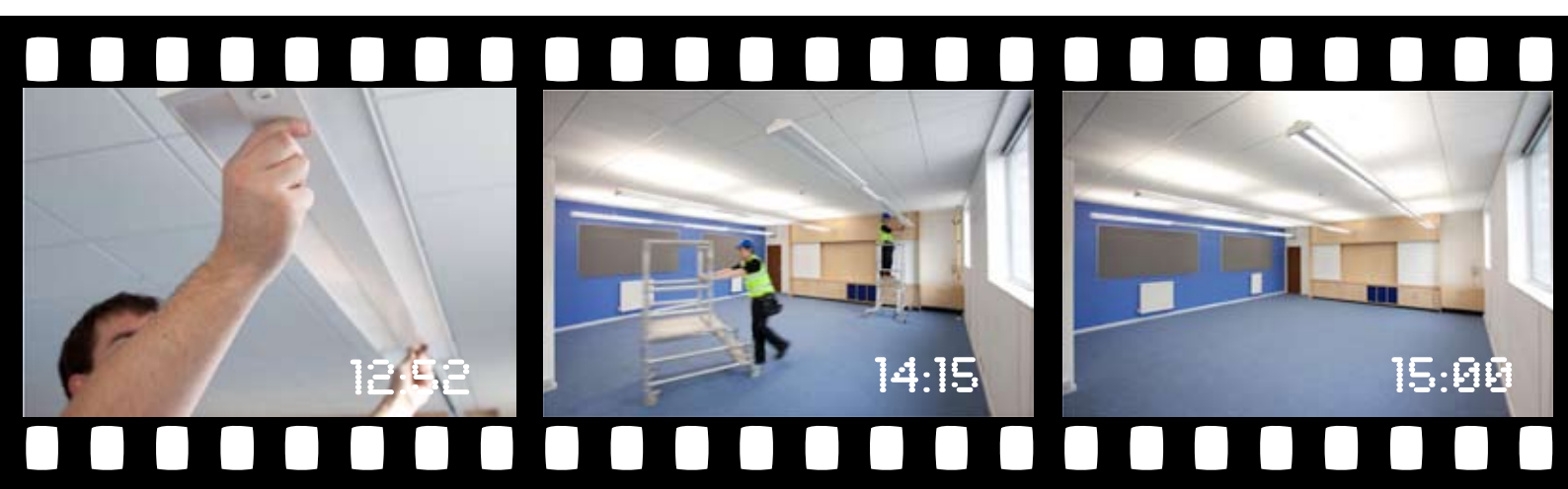
12:52 The luminaires are affixed to the track by means of fast lock.
