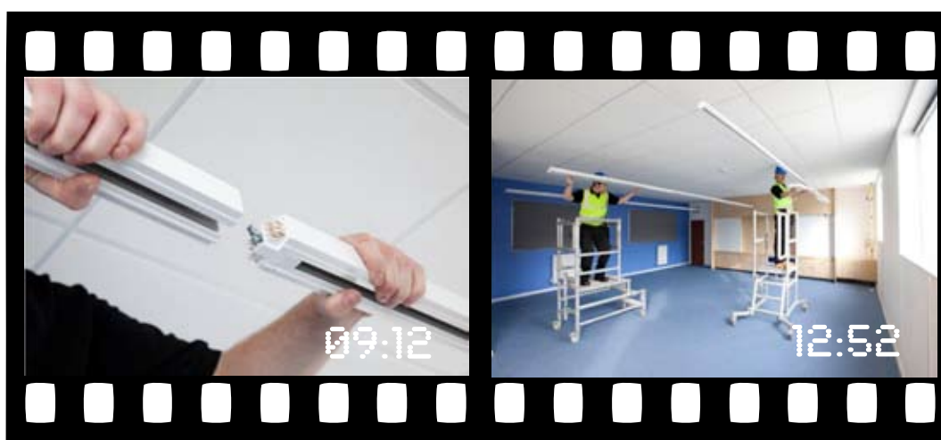
09:12 iTrack is easily suspended from the wire bracket and the second track length is assembled and secured with a screw fastener.
