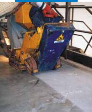
Preparation of the substrate by shot basting
