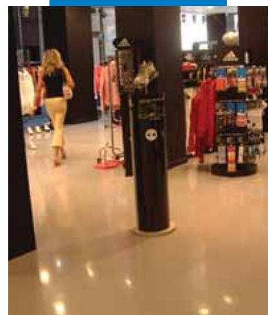
Floor made using Ultratop, then dressed using the self-levelling Mapefloor System 33
