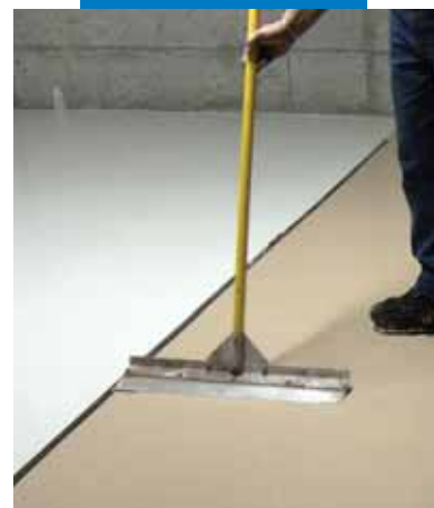
Smoothing Ultratop immediately after spreading
