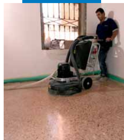
Final step of dry-polishing process of a floor made using Ultratop/Dynastone Color
