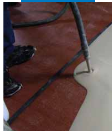
Mechanical application of Ultratop
