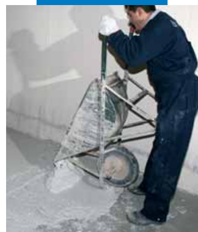
Spreading Ultratop and Dynastone Color mix
