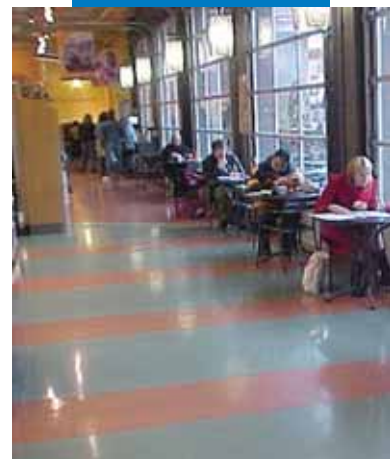
Two different shades of Ultratop followed by polishing operation
