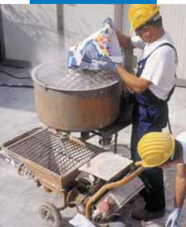
Mechanical preparation of the product before pumping
