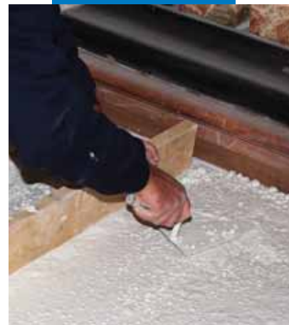
Flattening and compacting Ultratop mixed with Dynastone Color aggregates
