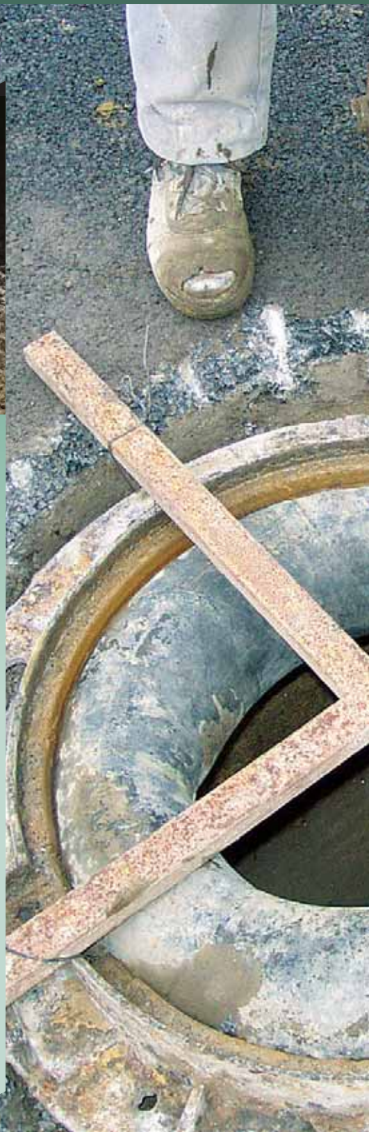
Road maintenance work - Chayenay sur Seine - France Repairing a man-hole using: MAPEGROUT SV
