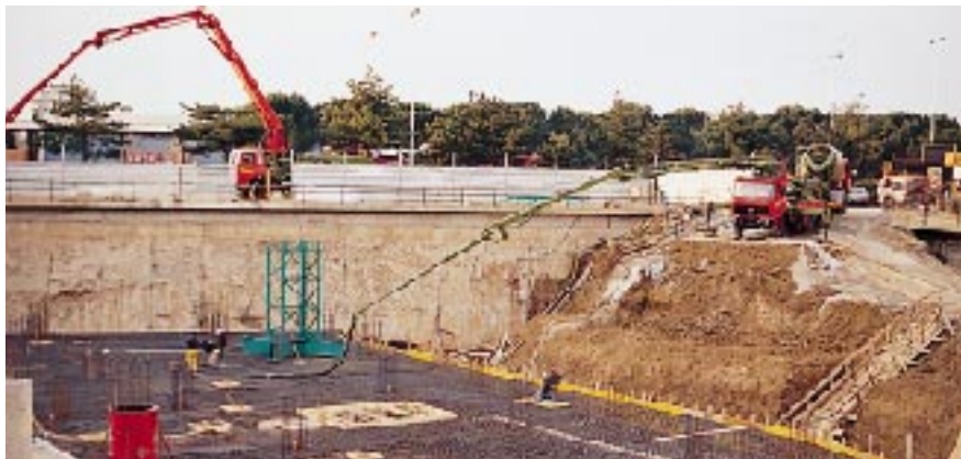
Casting a watertight foundation bed with concrete prepared with MAPEFLUID PZ500 admixture
