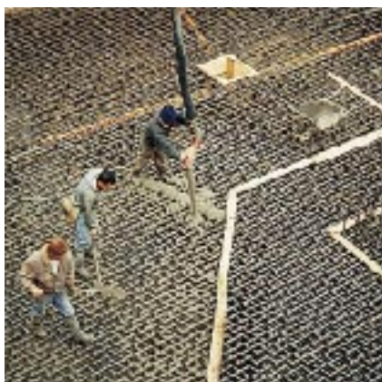
Detail of casting of foundation bed with superfluid concrete admixed with MAPEFLUID PZ500
