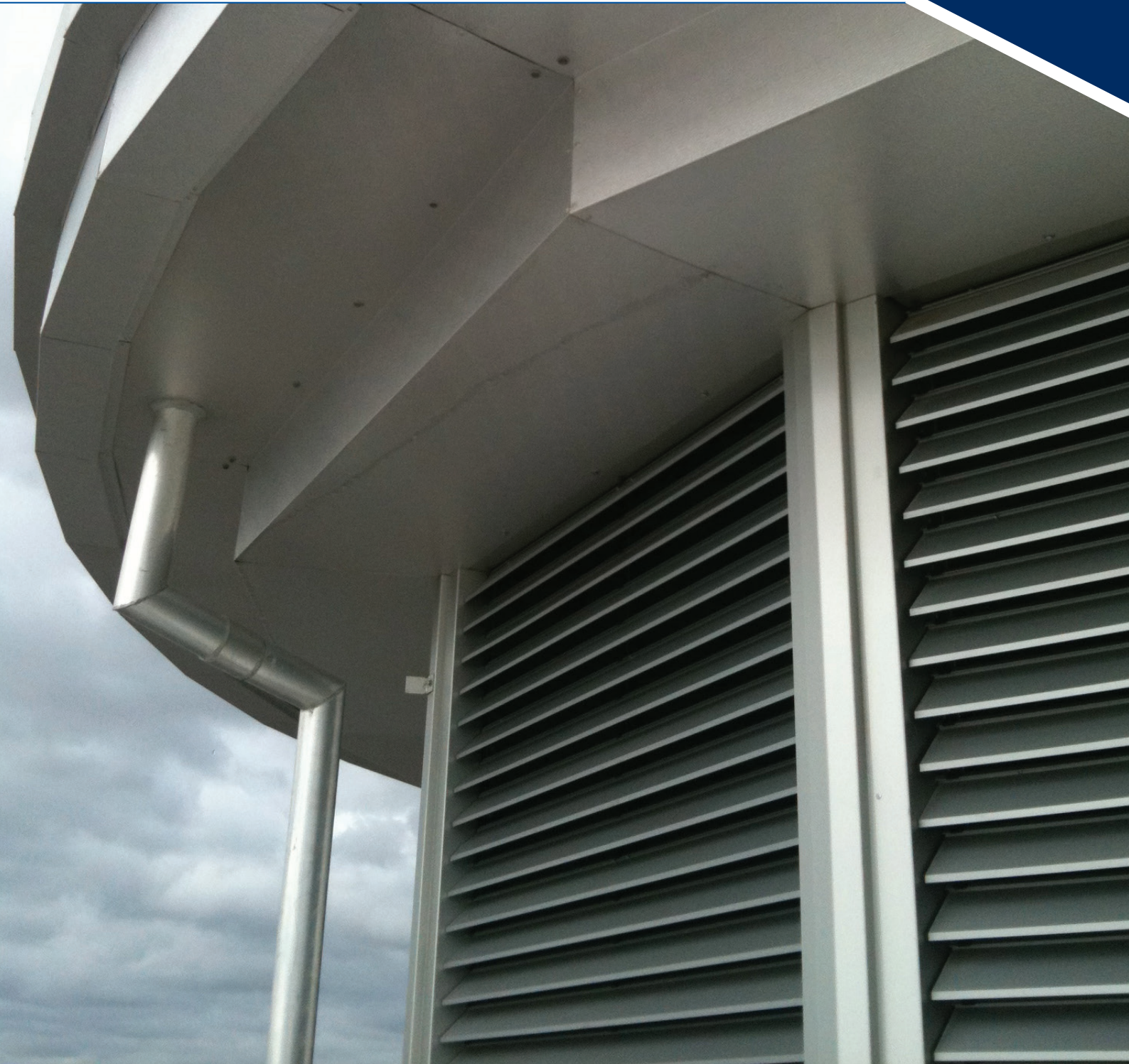
MAIN PICTURE: SYSTEM 75 LOUVRES, WESTON- SUPER-MARE PIER
