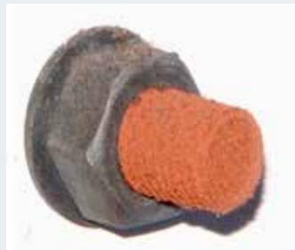
Fastener that has been affected by red rust.
