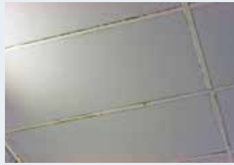
An acoustic ceiling (on the left) where the grid has corroded due to choice of an incorrect choice. A Connect C4 grid of homogeneous, acid resistant steel would not have been affected, as seen in the picture to the right.
