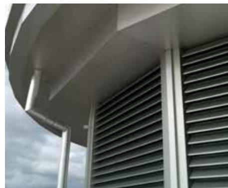
Lareine 75mm fixed louvre system available for screening or performance purposes
