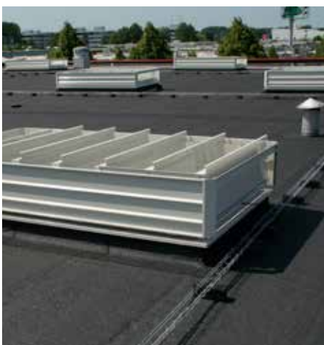
Lareine louvered smoke ventilators are available with insulated aluminium, glass or Isolux louvres, controlled electrically or via compressed air
