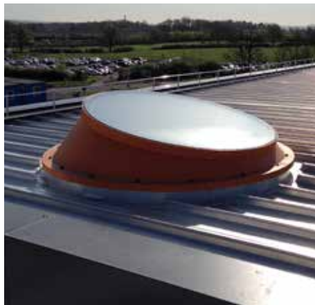
Circular rooflights, Worcester Hospital
