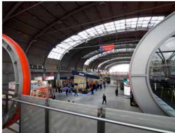
Exhibition hall daylighting
