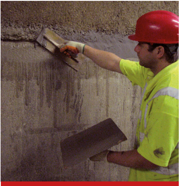
Construction joint repair using Triton Fillet Seal.
