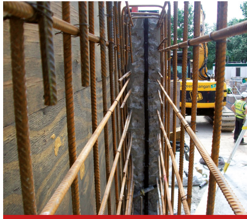
1. Chase Cast in centre of wall section/joint section. Approximately 20mm x 15mm
