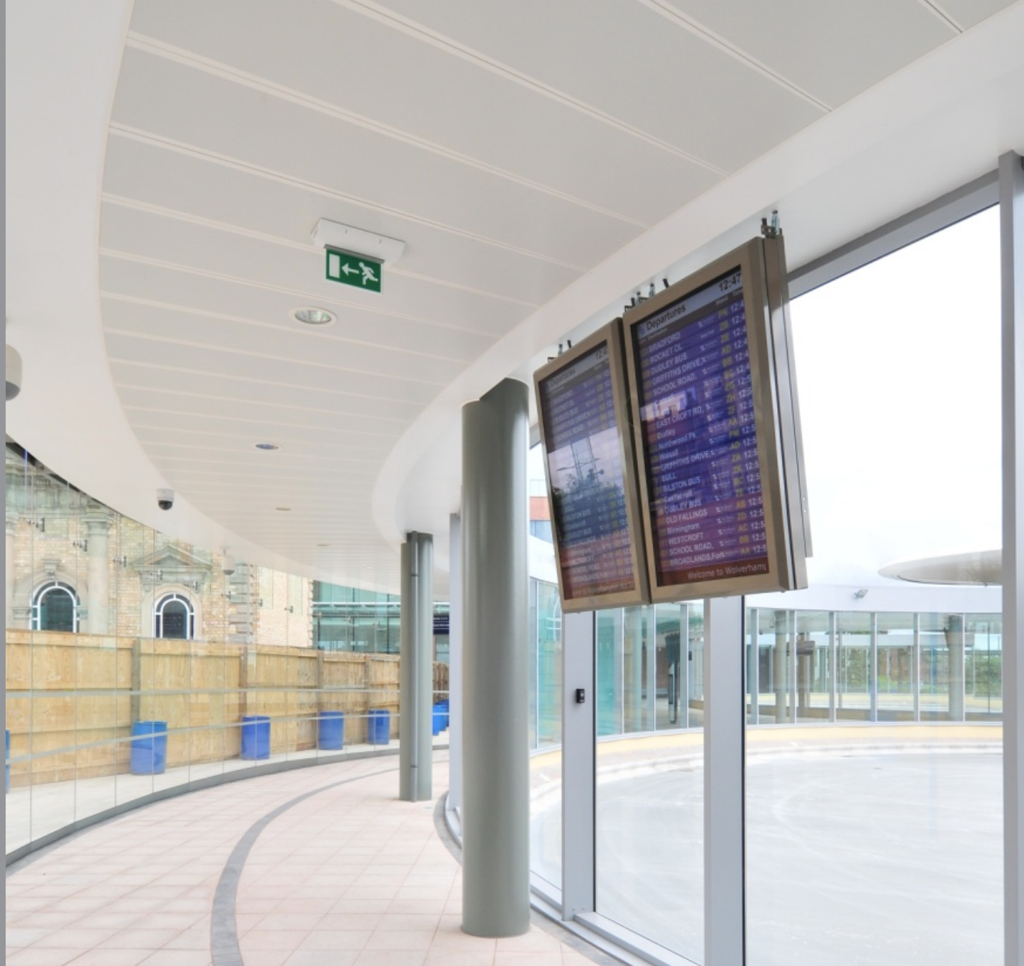
Wolverhampton Bus Garage (UK) Square Edge Microperforated Trapezoidal Metal Planks with fleece
