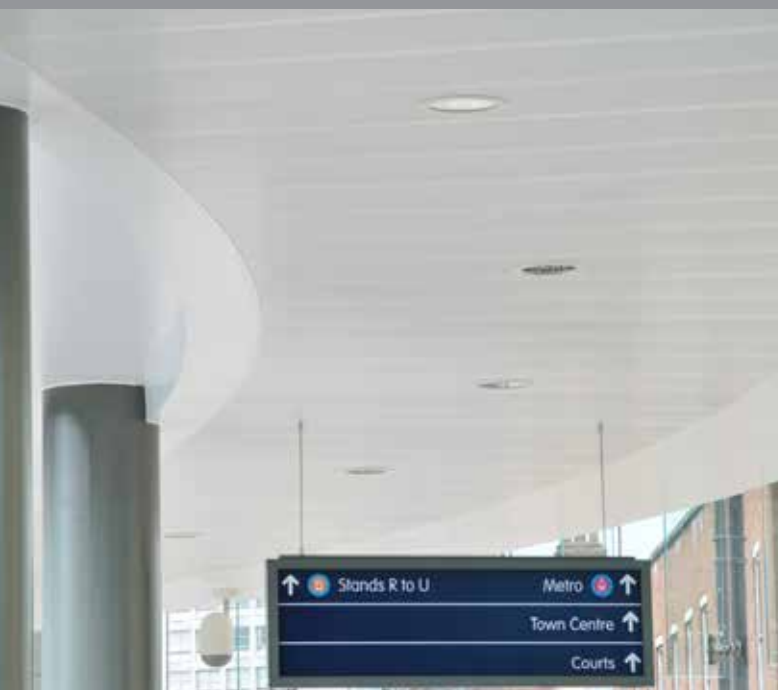
Wolverhampton Bus Garage (UK) Square Edge Microperforated Trapezoidal Metal Planks with fleece
