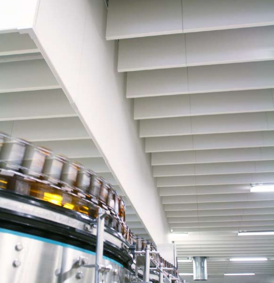
An open system with vertical baffles is a good alternative when a wall to wall ceiling cannot be used.
